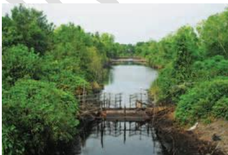
Figure 3-4: Successive ditch blocks made of wood and soil bags in a medium-width canal in Central Kalimantan.
