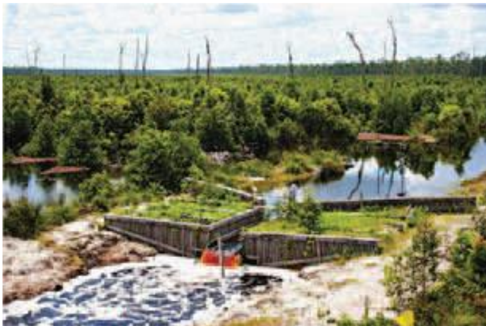
Figure 3-1: Dam constructed to systematically block a former logging canal to restore peat swamp water levels.
