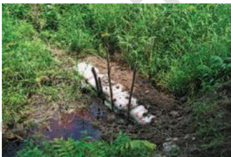
Figure 3-3: Small ditch blocked with sandbags and soil
