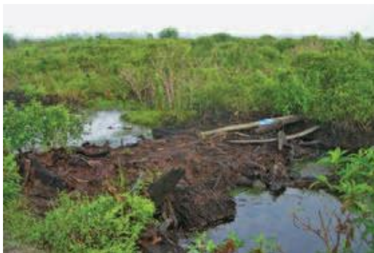
Figure 3-2: Small ditch blocked with peat dam.
