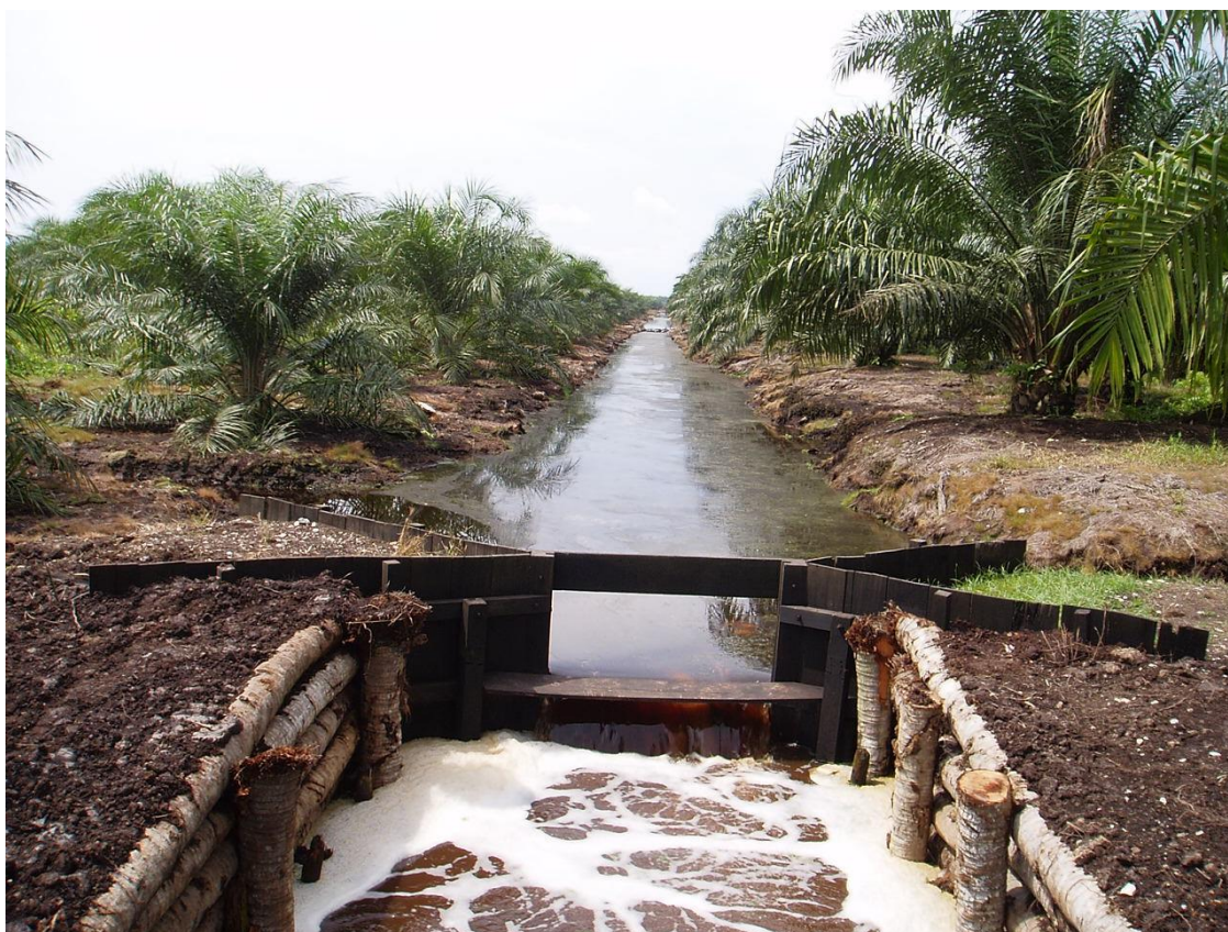
Figure 3-5: More sophisticated (but still low cost) structures on collection drains can be constructed with earth fill and wooden boards (example from United Plantations, Malaysia)
