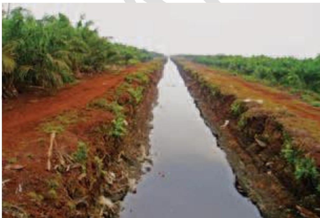
Figure 3-8: Over-drainage in main drain in a peat dome area during dry seasons may result in high CO 2 emissions, subsidence rates, increased risk of accidental fires, as well as significantly reduced yields.
