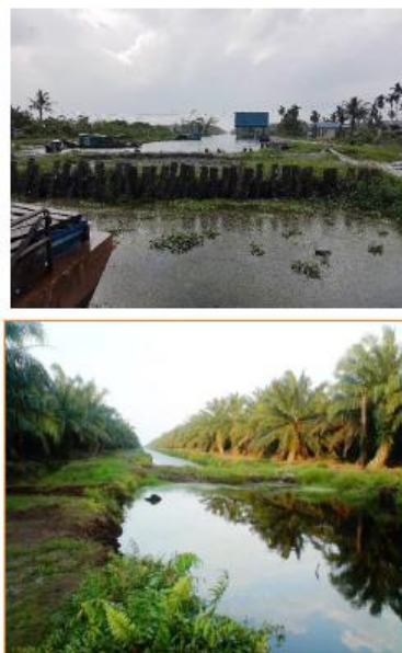
Figure 3-17: A key part of implementation of the water management system is the division of the plantation into different water management zones – with relatively constant water level in each zone
