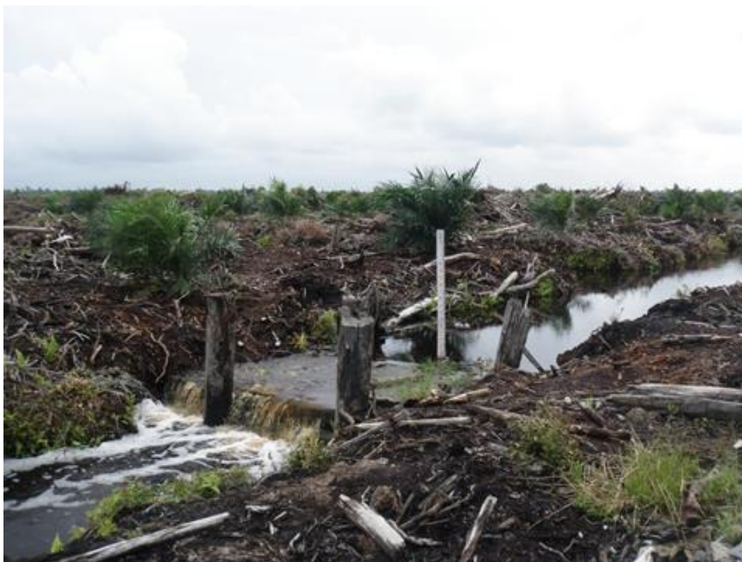
Figure 3-4: water control structures do not need to be expensive structures and can be simply constructed with wood or sand bags.
