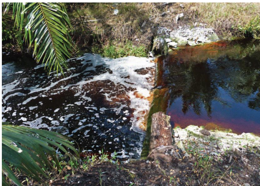
Figure 7-4: One weir installed at every 20 cm drop in water level to enable water retention along collection drains
