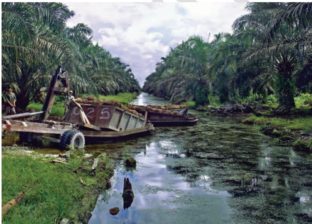
Figure 3-12: Following the contours and setting high water levels along collection drain in Woodman estate in Bintulu, Sarawak enables FFB to be transported by barge pulled by a small boat with a 15hp engine.
